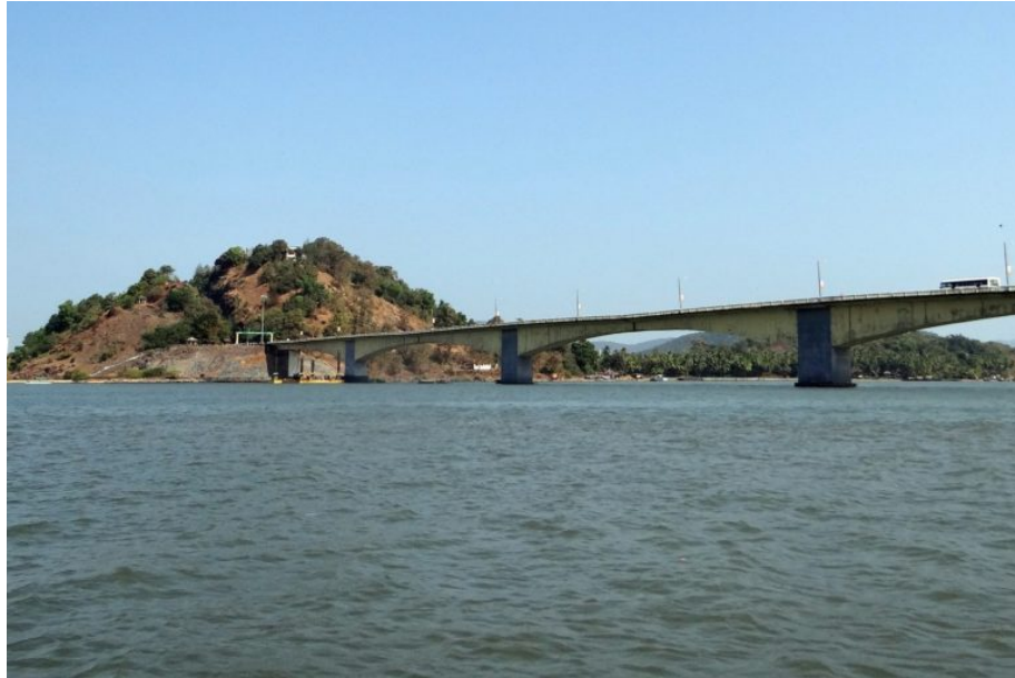
A bridge on the Kali river. Photo from Sarangib/Pixabay.
